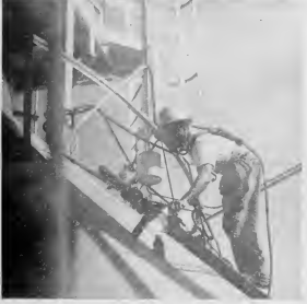
Cyril Fitz is not 300 feet in the air, painting the Cal Plant's steel structure. He is 300 feet in the air, painting the Cal Plant's steel structure. He is 300 feet in the air, painting the Cal Plant's steel structure.
